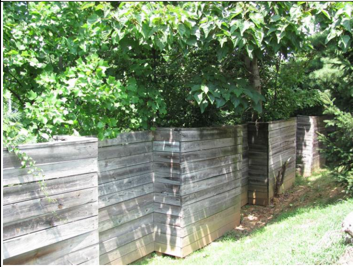
Photo #11: Wood retaining walls
