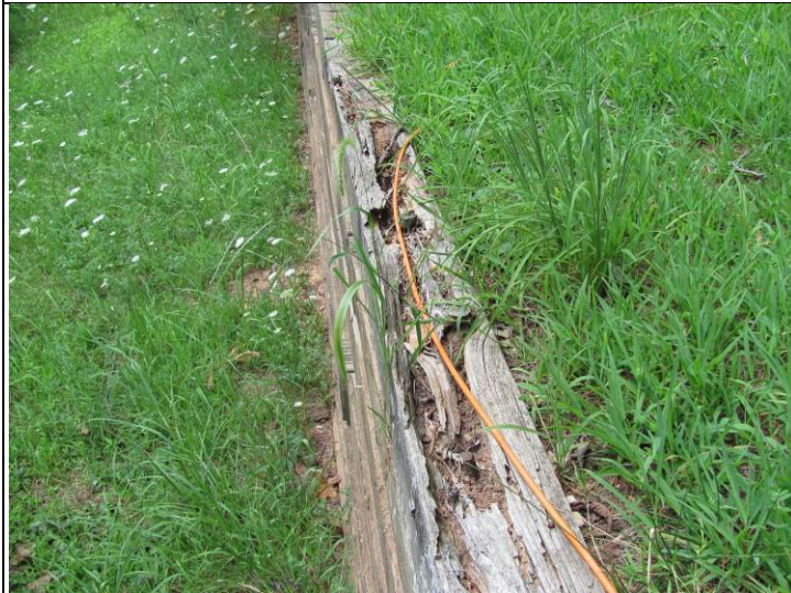
Photo #14: Wood retaining walls
