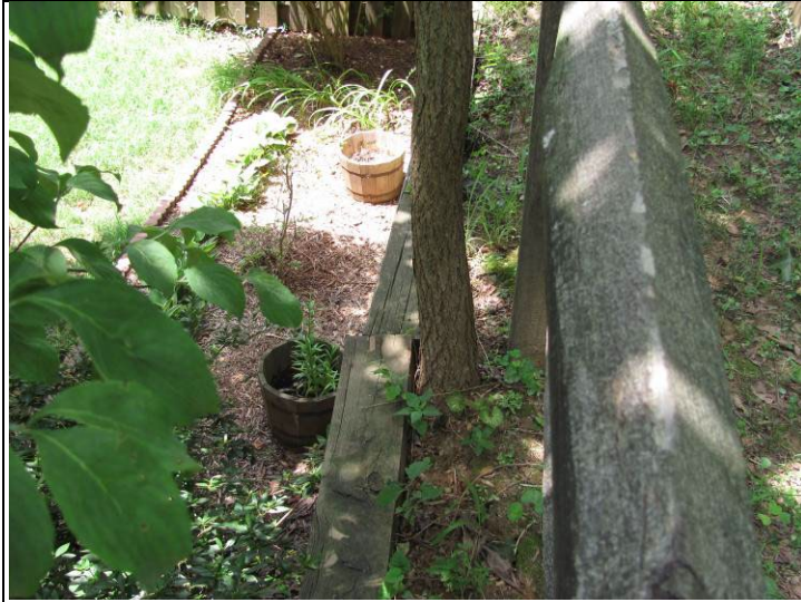
Photo #16: Wood retaining walls
