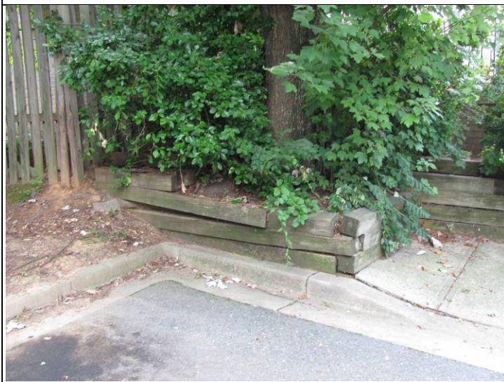
Photo #18: Wood retaining walls
