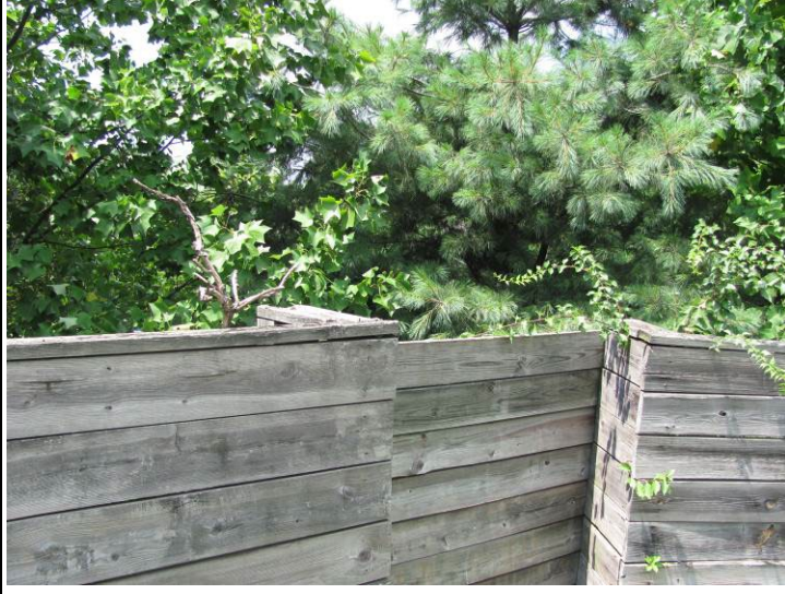
Photo #10: Wood retaining walls
