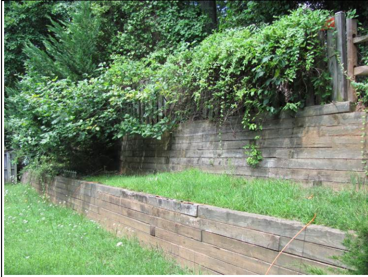
Photo #13: Wood retaining walls
