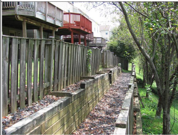
Photo #21: Wood fence and wood retaining walls
