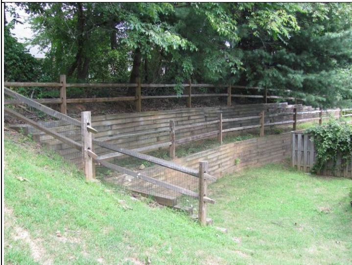
Photo #17: Wood retaining walls and fence
