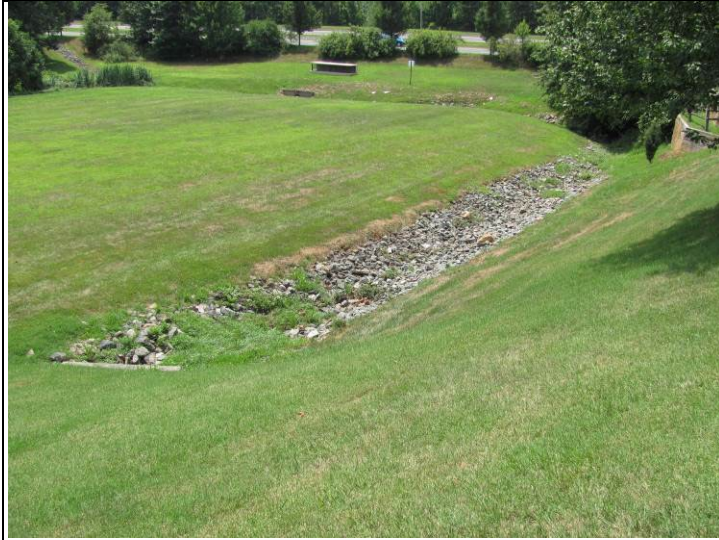
Photo #19: Rip rap area covered under storm management
