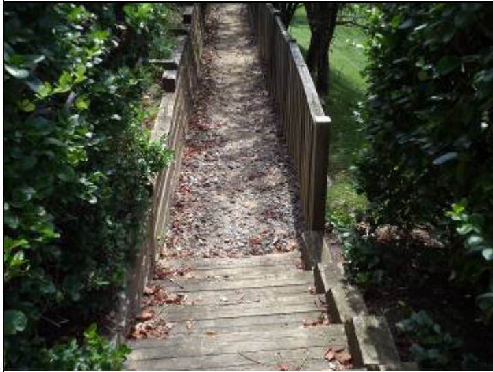
Photo #50: There is a graveled walk along the drainage field. We recommend additional gravel be added. This would be considered a maintenance issue.
