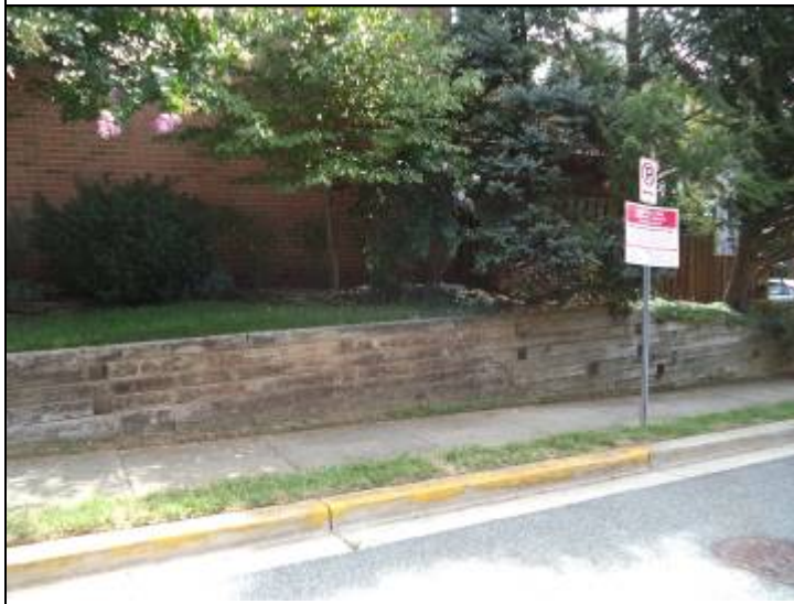
Photo #39: Site wood retaining wall
