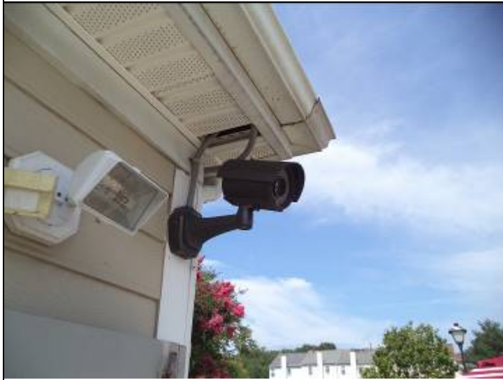
Photo #14: New camera systems have been added to the pool house building.
