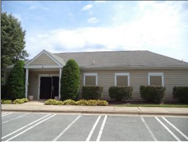
Photo #1: Pool house building and roof
