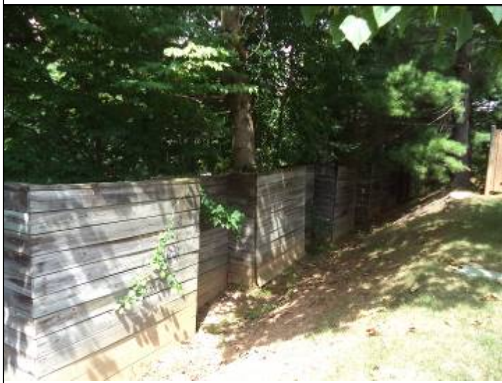
Photo #36: Site wood retaining wall
