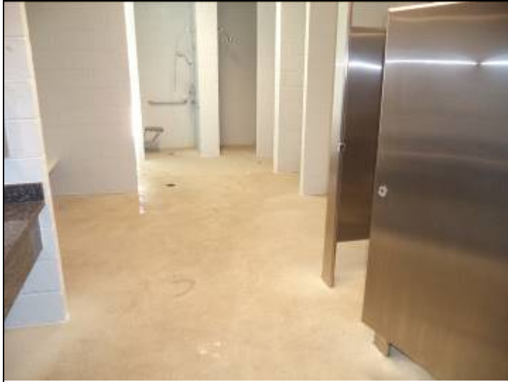
Photo #10: Pool house men's room
