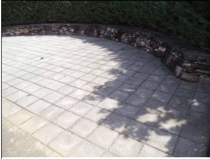
Photo #28: Concrete paver area with stone retaining wall
