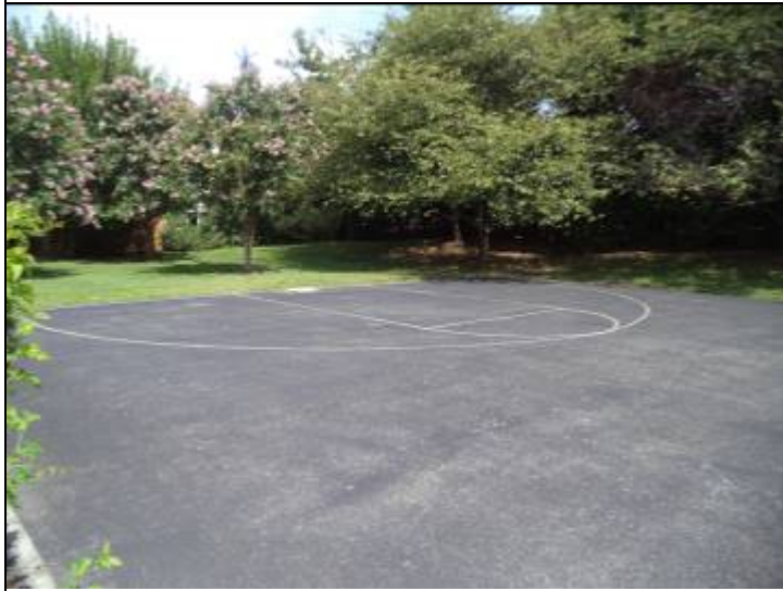
Photo #32: Other than cosmetically removing the asphalt surface, we can recommend possibly using this for additional services.
