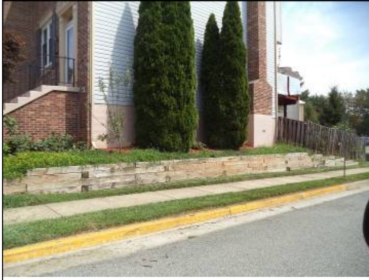
Photo #49: Site wood retaining wall
