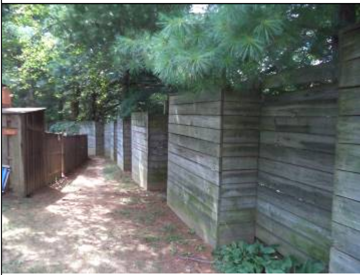
Photo #42: Site wood retaining wall
