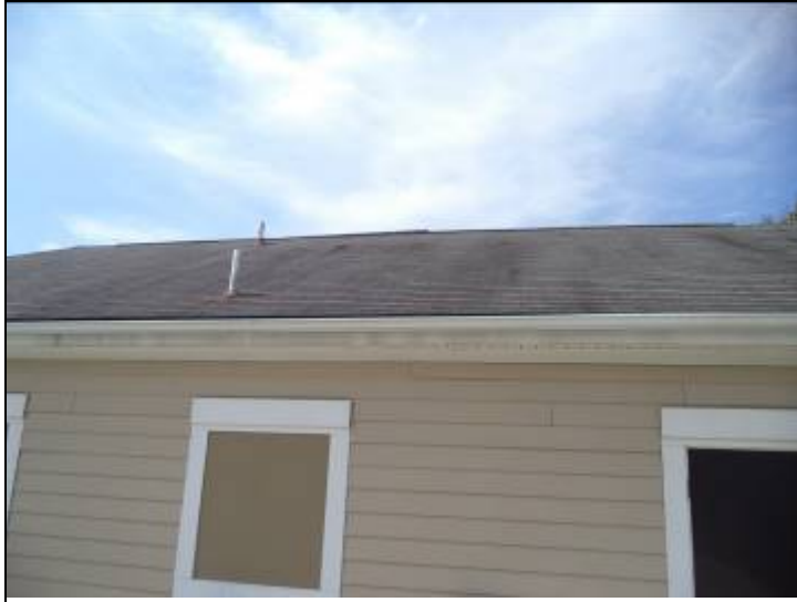
Photo #16: Pool house roof system
